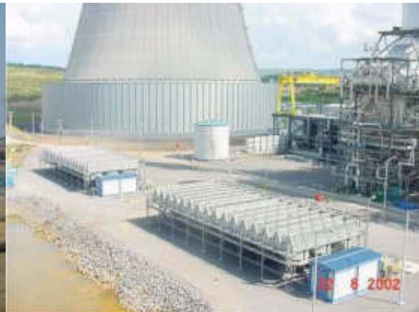
Figure 4.5 Photograph showing a power station with the water-to-air heat exchangers of the Stack-in-Tower system of indirect dry cooling technology
