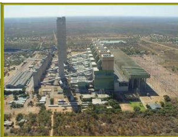
Figure 4.9 Photograph showing a power station with direct dry cooling technology
